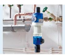
Application For the protection of drinking water installations against corrosion as per DIN 1988. The pressure reducer reduces the inlet pressure to an even, system-specific pressure in order to protect the installation and to ensure economical water consumption. Water filters help to keep pollutants such as rust particles and sand grains from reaching the domestic water installation and thus protect valves, machines, flow heaters, etc. from malfunctions caused by pollution.
